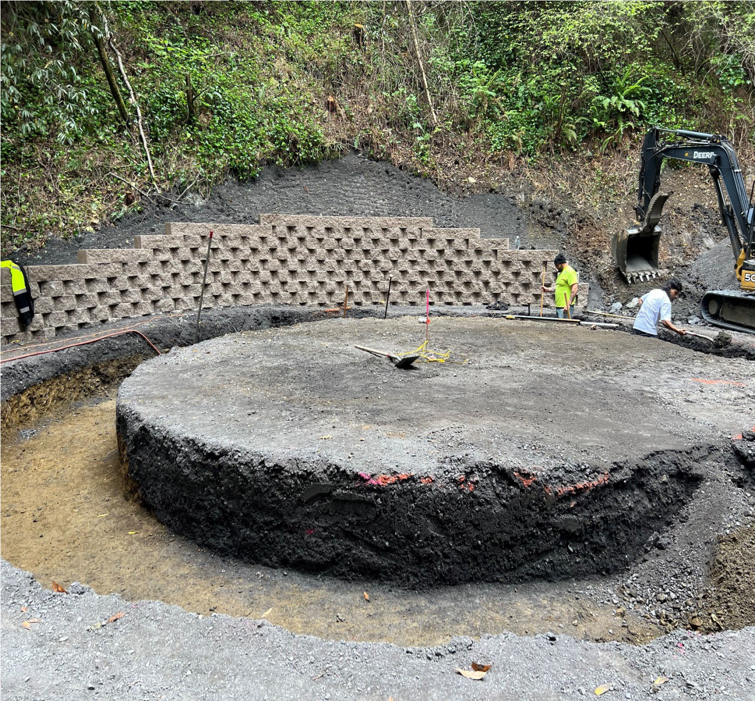
Retaining Wall and Tank Ring Prep 4/24/2024.
